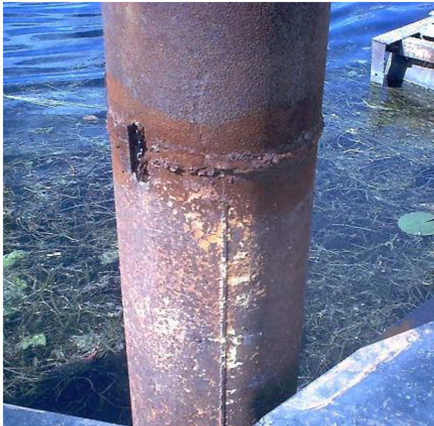
Figure (2-2) Uniform Corrosion [10]
